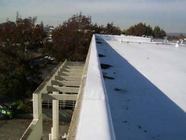
The perimeter concrete walls were roofed with the same membrane that was installed over the entire roof surface. The sheets were fully adhered using water based adhesives.
