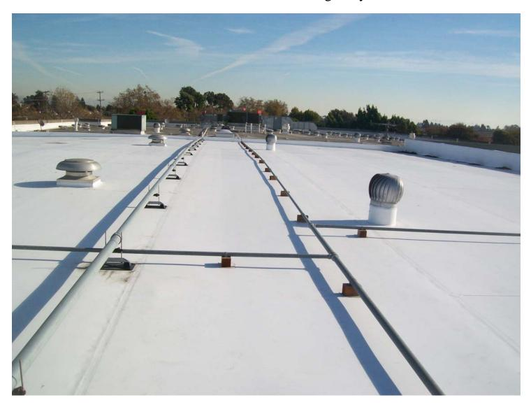
The existing capsheet surfaced Built Up Roof was overlaid with EPS Fanfold insulation and Firestone .060 mil polyester reinforced TPO single ply. In addition to replacing the wood sleepers under the conduit, the large gas line was set on roller supports to allow for expansion and contraction.
