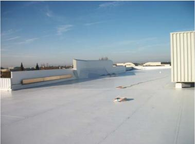
The EIFS system above the entry was sealed with a polyester reinforced emulsion system followed by the application of white acrylic coating applied at 3 gal. per 100 sq ft.
