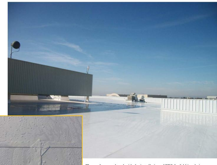
The roof was replaced with the installation of EPS fanfold insulation installed over the existing capsheet surface followed by the installation of Firestone .060 mil polyester reinforced TPO single ply.
