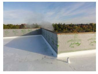
The concrete perimeter walls were clad with AEP Span Kynar Coated Metal panels with a synthetic self adhered underlayment, PTDF wood nailer and metal cap flashing with drive cleat seams that do not require sealant.
